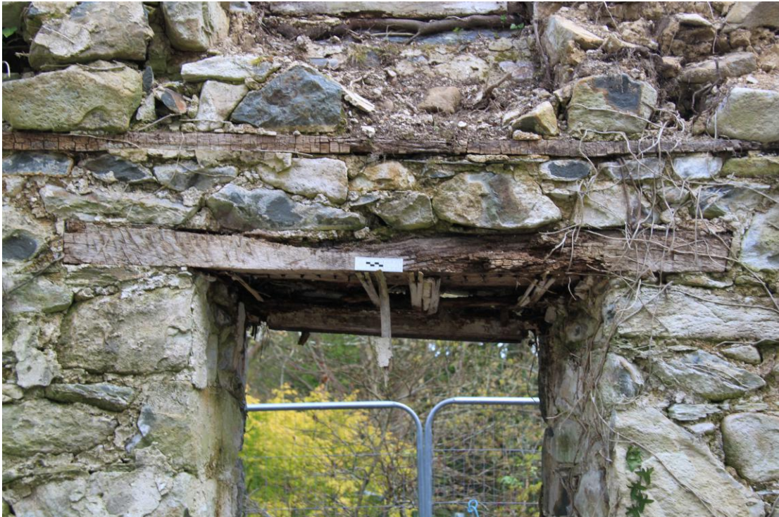
Plate 16 - AD010-BR-016 - Oak window lintel, internal, north wall.
