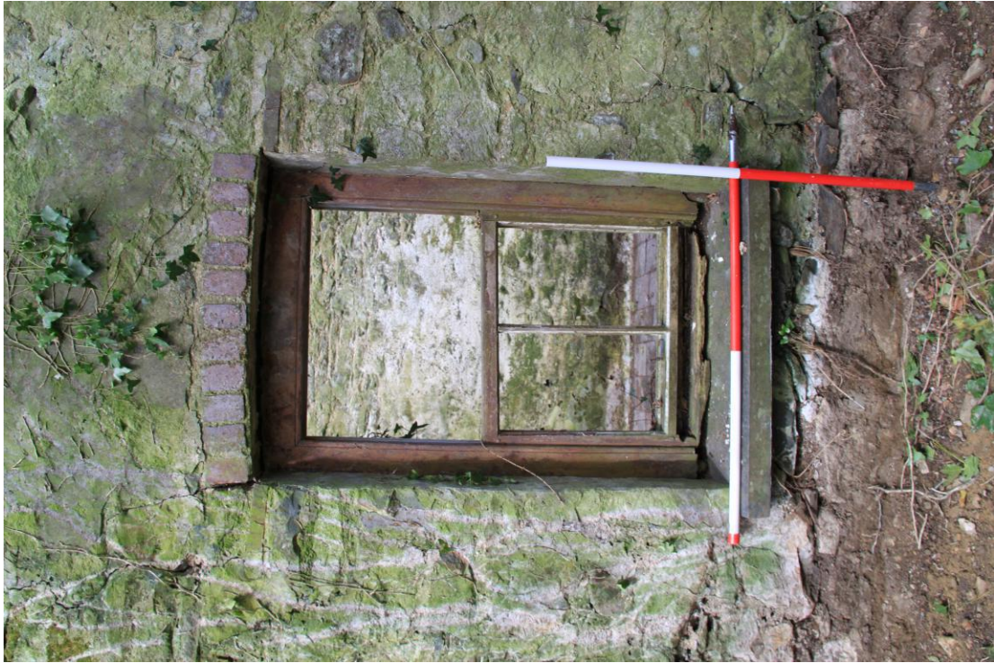
Plate 47 - AD010-BR-047 - Remains of four light box sash window, Extension A east elevation.
