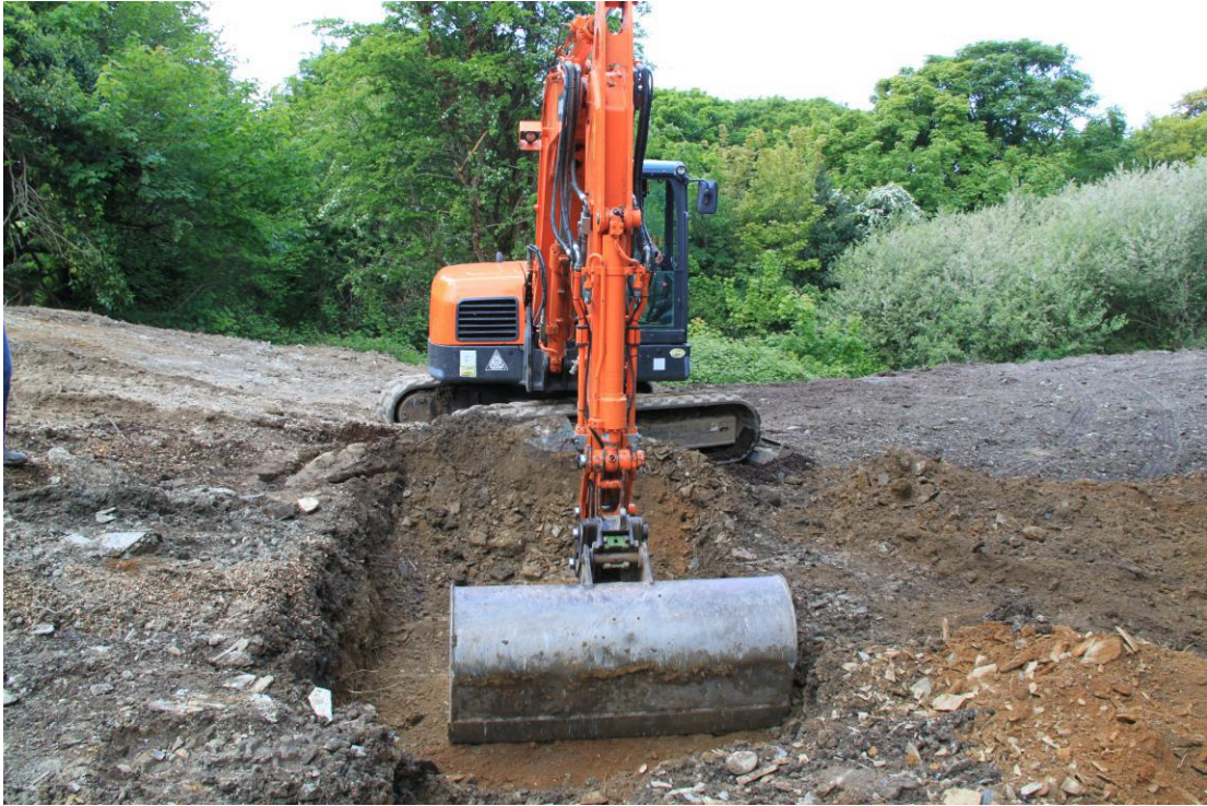
Plate 66 - AD010-D3-019 - Excavation of septic tank pit.
