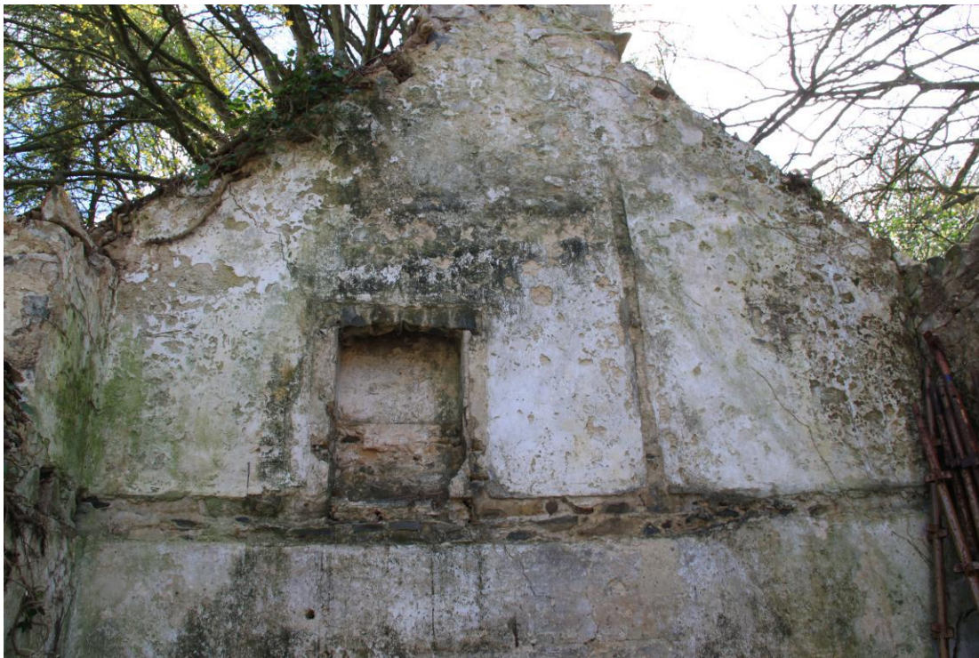
Plate 25 - AD010-BR-025 - First floor fireplace, internal east wall, Former Coach House. N.B. Partition division mark to plaster.
