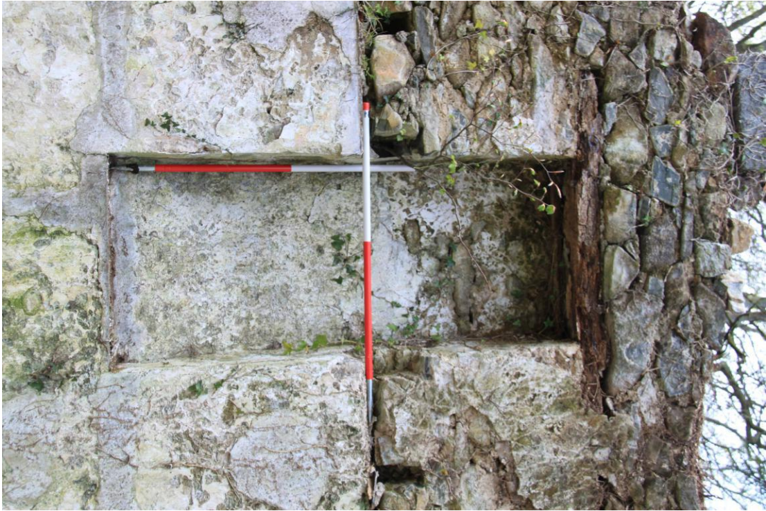
Plate 15 - AD010-BR-015 - Hay feeder shoot, internal, south wall.
