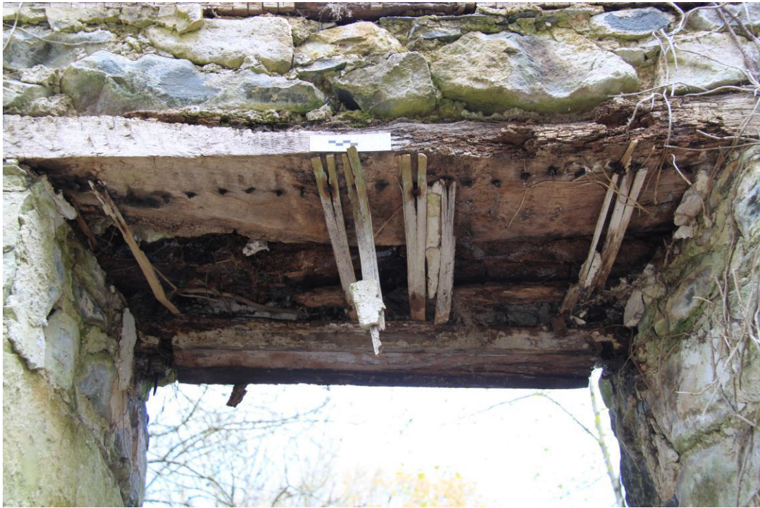
Plate 17 - AD010-BR-017 - Oak window lintel, internal, north wall.
