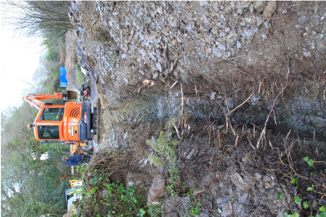
Plate 55 - AD010-D1-008 - Service trench 1 cutting through disused leat.
