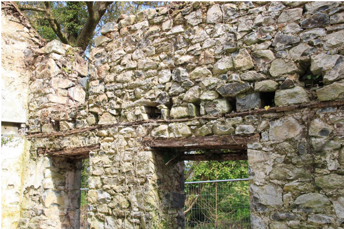
Plate 18 - AD010-BR-018 - Joist sockets, internal, north wall.
