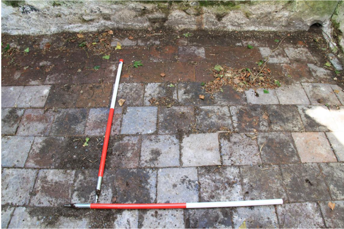
Plate 37 - AD010-BR-037 - Quarry tile floor to Extension A.
